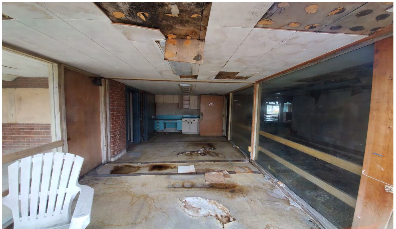
PHOTOGRAPH 26 Interior view of former True Value Hardware store building.
