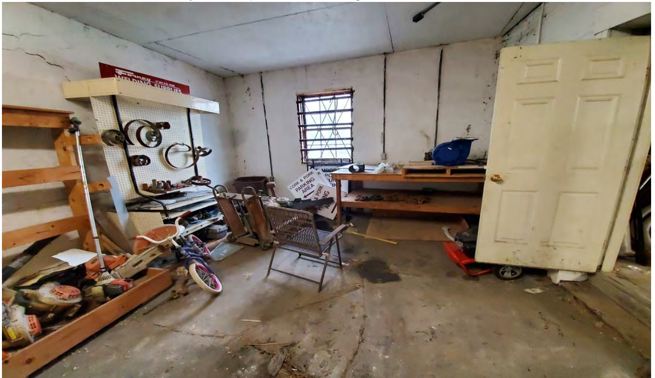
PHOTOGRAPH 18. Interior view of eastern side of former True Value rental building.
