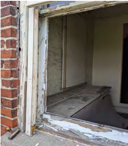
Samples 2-01 to 2-03 (ACM - Gray Window Glazing)
