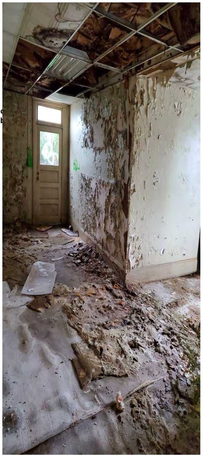
PHOTOGRAPH 24. Interior view of former Nettleton Planing Mill office building.
