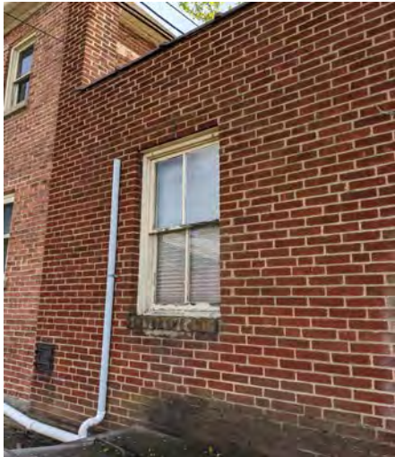
Sample 2-P-08 (LBP – Cream Exterior Window Sash)
