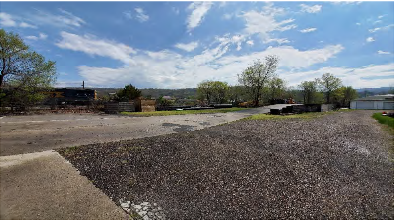
PHOTOGRAPH 13. Rear of True Value building. Former Nettleton Planing Mill building slab and loading dock. Railroad in background.
