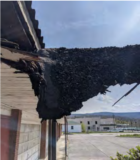
Samples 3-25 to 3-27 (ACM – Original Asphalt Roofing)
