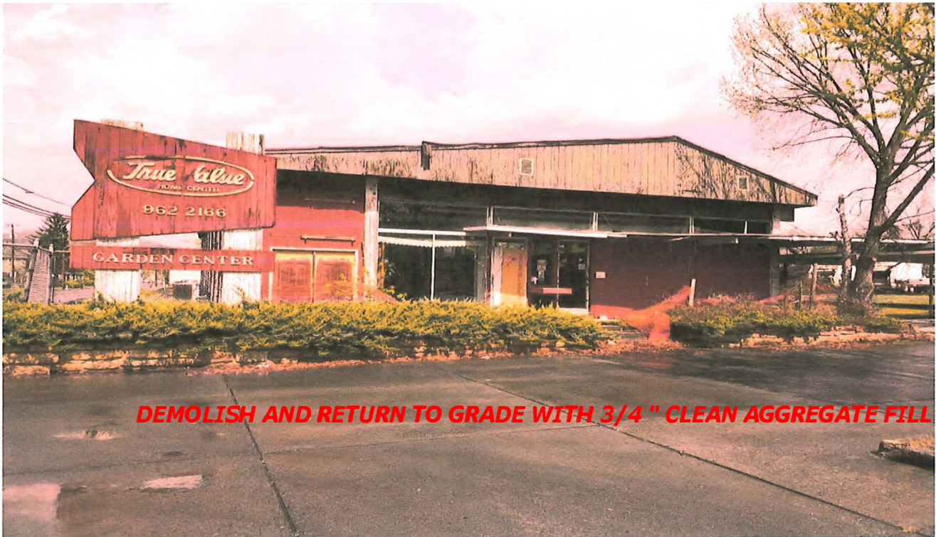
PHOTOGRAPH 1. Subject property. Former True Value Hardware store building. ( south face )
