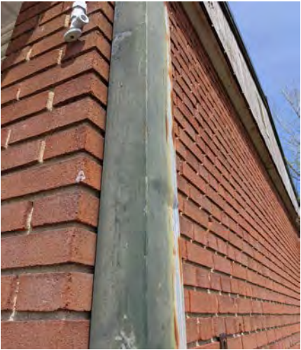
Sample 4-P-03 (LBP – Green Roof Drain Paint)
