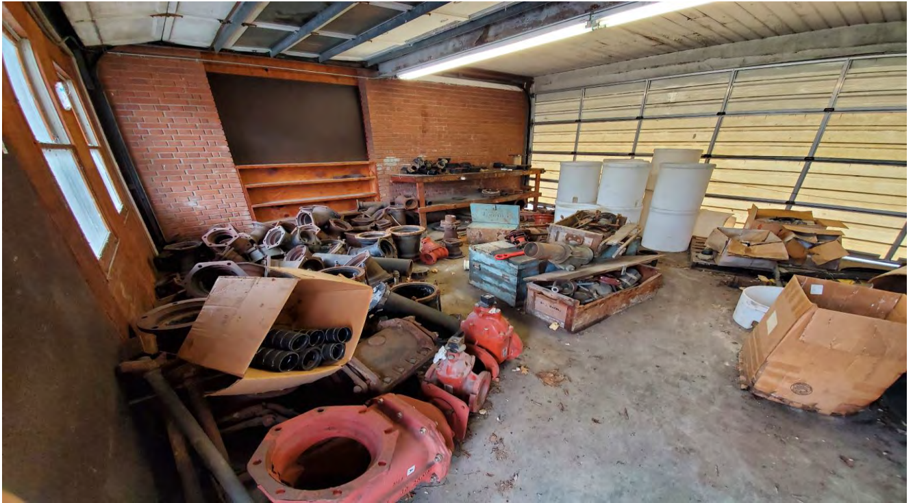
PHOTOGRAPH 19. Interior view of former True Value garage building. Currently used for City water department for storage.
