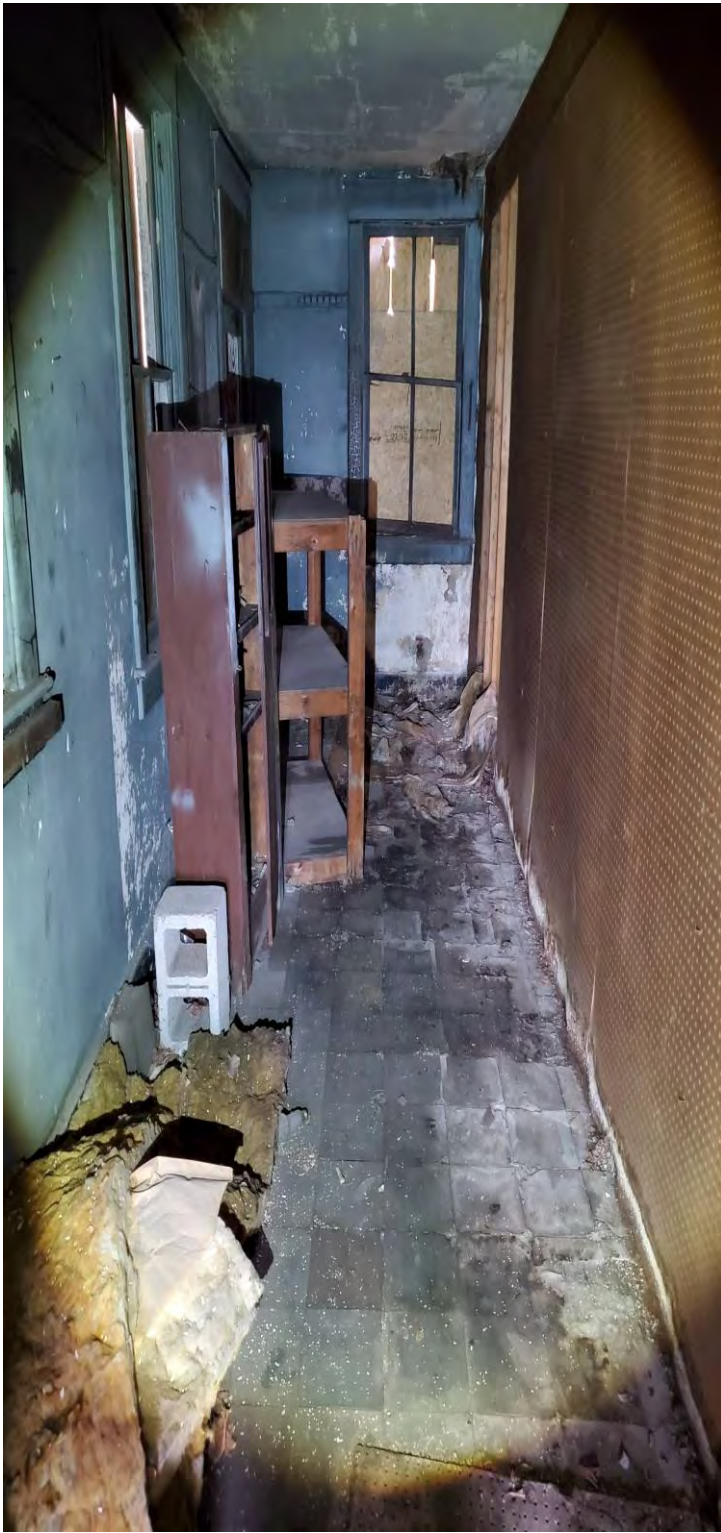
PHOTOGRAPH 23. Interior view of former Nettleton Planing Mill office building.
