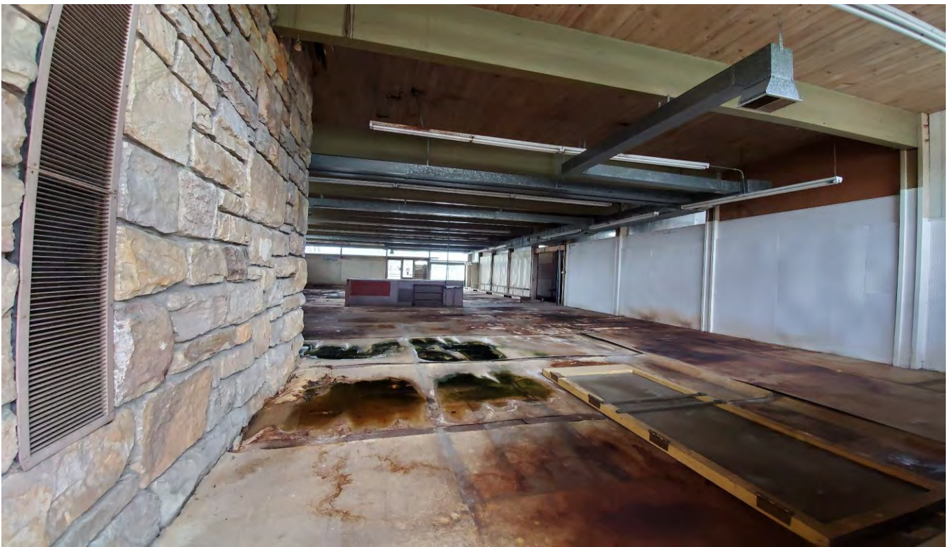
PHOTOGRAPH 25. Interior view of former True Value Hardware store building.
